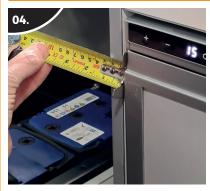
Position the fridge so that it is centred with specified ventilation gaps, be careful to keep the fridge upright and avoid trapping any wires.
